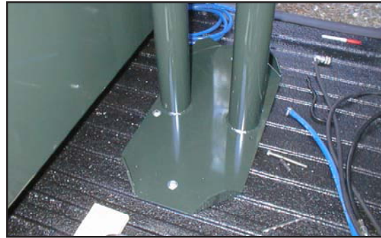
Figure 9. Mount Bracket Parallel to Recovery Tank For Accessibility
